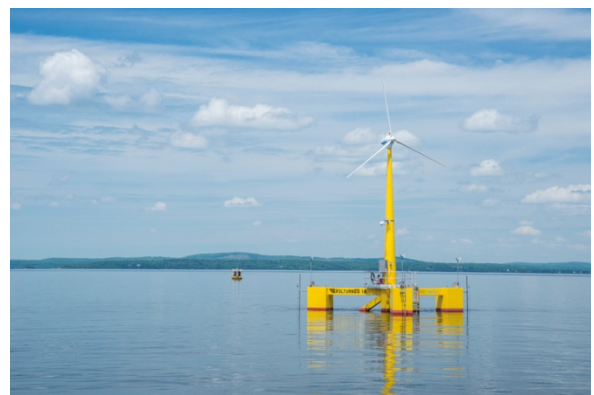
Image of the University of Maine's VoluturnUS 1:8 scale platform .
